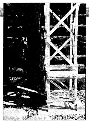
Wood you put up a tower like this one? Excuse the pun, but it applies perfectly to these photographs. Douglas Bainbridge, NØHPK, assembled a 72-foot tower made entirely of Douglas fir and held together with nails and epoxy adhesive. From a distance it looks like any steel tower (right). Only when you're up close (above) do you realize that it is made of wood. Despite the load from his 2-element, 15 and 17 meter quad antenna, the tower has withstood wind gusts above 70 MPH.
